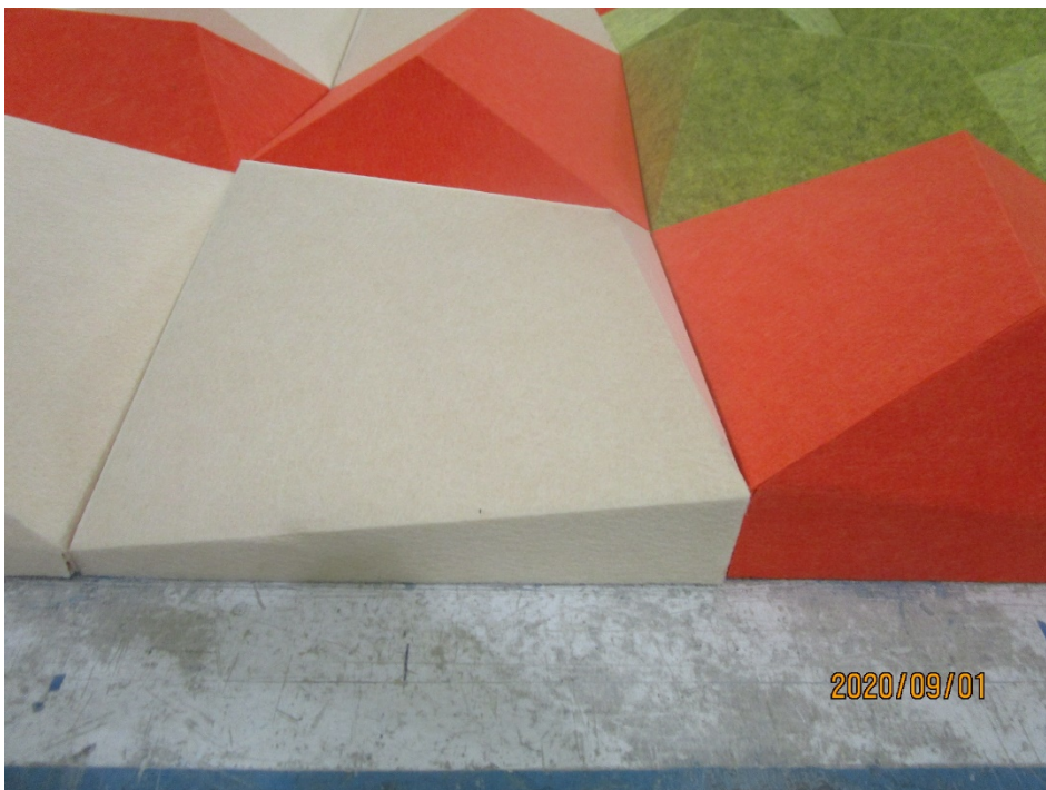
Figure 4 – Relative orientation of adjacent panels as installed
